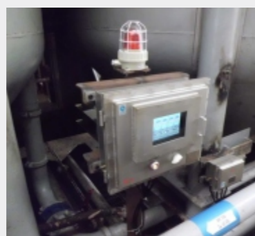
现地仪安装图片 Instrument installation drawing
