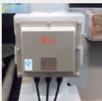
防爆接线盒现场 Explosion-proof junction box
